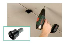
A special drywall interior fitting bit with pressed depth stop is used in order to correctly sink the screw and avoid damage to the board when screwing it into position. The most well-known screw- driver for this purpose is a size 2 Phillips bit. The screw sequence is important in order to prevent the boards from deforming; however, it can be stipulated differently depending on the manufacturer.
