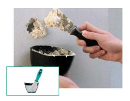
With regards to two-layer planking, this also has validity for the bottom board layer. A second finer coating of filler can be applied after drying, so as to achieve a better surface result.
