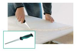
Larger holes or cut-outs are marked and can then be cut out using a hand jigsaw. Pre-drilling is not necessary, due to the bevelled and partially ground point of the saw blade.
