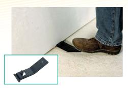
In order to ensure that the plasterboards on the wall have the necessary distance from the floor, they must be lifted slightly and held in the correct position. This requires little effort with the help of the board lifter and your foot.
