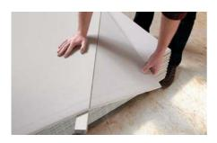
The plasterboard is marked along the cutting aid with the knife and then carefully broken over a sharp edge. The backing board can then be cut through, if necessary.
