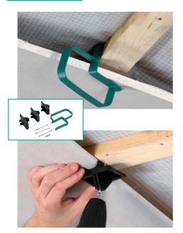
It is possible to attach boards to ceilings and pitches without the assistance of anyone else. The boards are fixed using the plastic fixing holders, the supplied screws and a metal clamp. The holders are removed and can then be reused for other boards.
